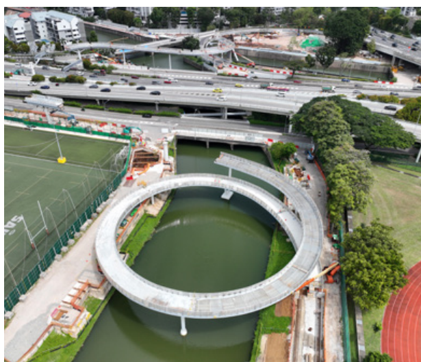
Aerial view of the elevated pedestrian and cycling bridge under construction.
